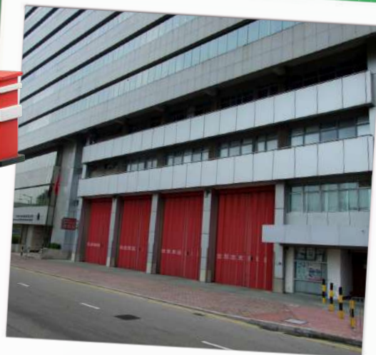
Tsim Tung Fire Station
